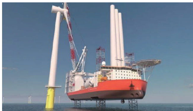
Figure 1. Jack-up Barge and Wind Turbine Installation. (Søfart, 2020)
